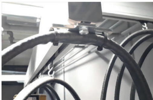
Example of an end stop with a strap.
