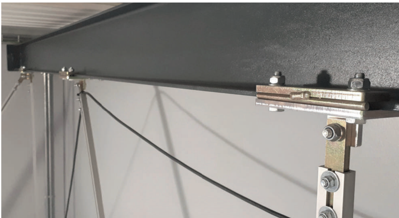
IPE bracket mounted with a Uni-suspension.
